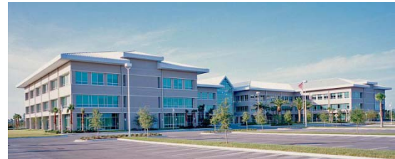
FCCI Headquarters and Florida Regional Office Sarasota, Fla.
